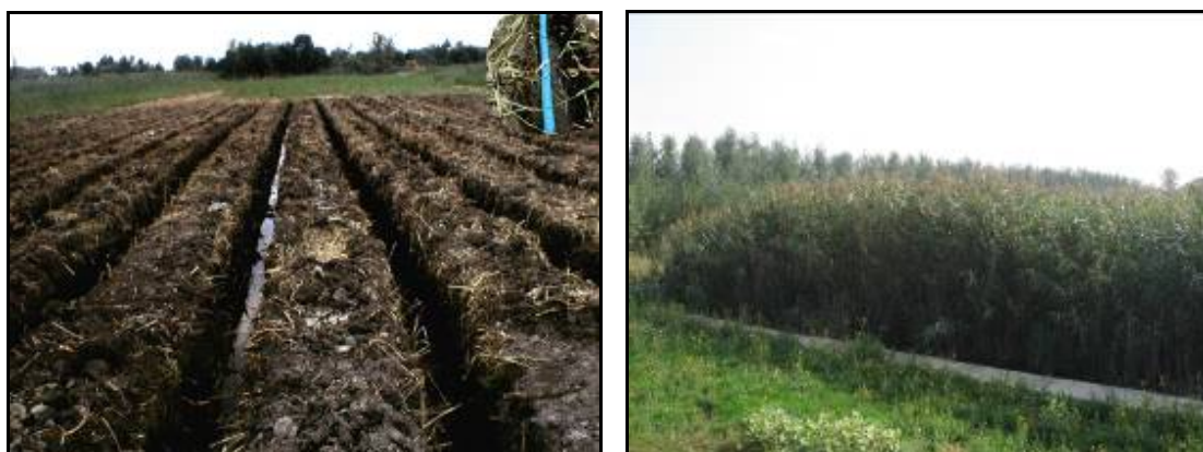
Figure 2. CWS in construction (2004) and after several years of operation (2008)
