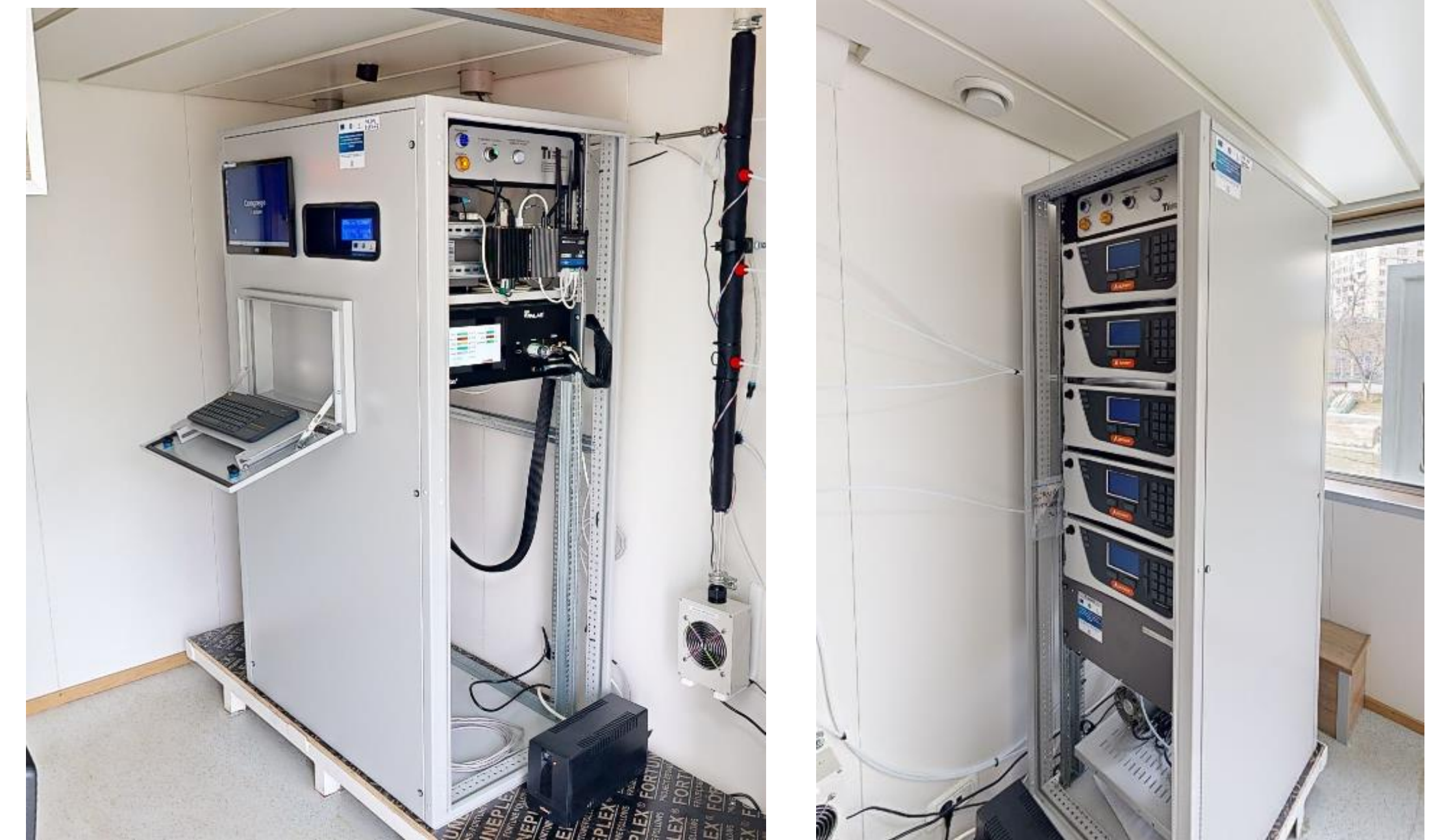
Figure 2. The System for air quality monitoring on board the REXDAN research vessel.
